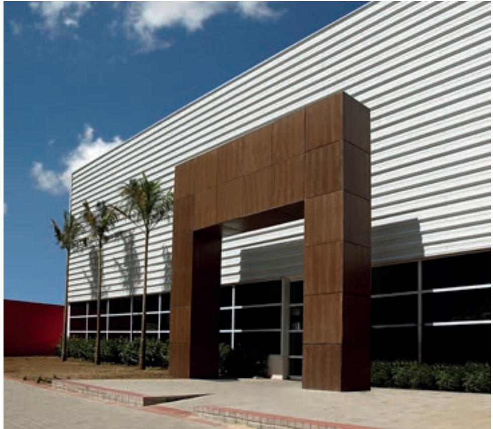
Application of the fiber-cement cladding panel Eterplac Wood
