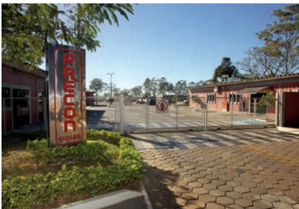
Precon Goiás Plant in Goiás
